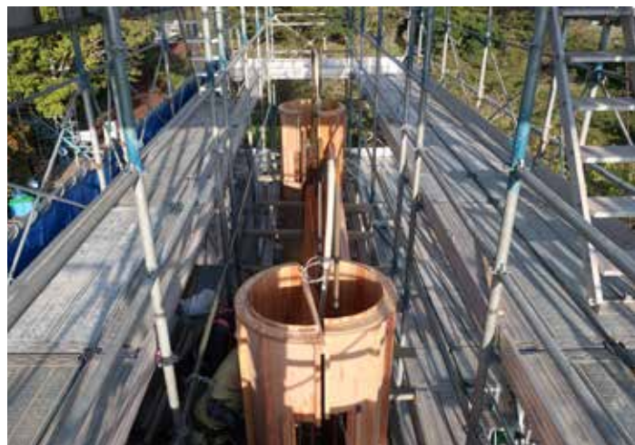
貫木部型枠建込
